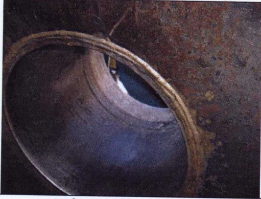
man way attachment weld
