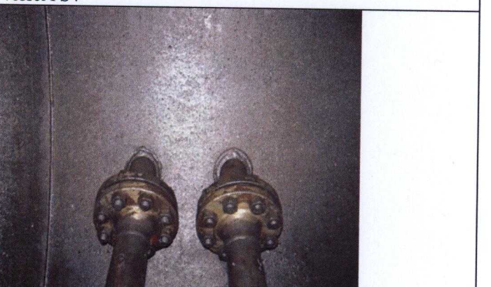
nozzle attachment welds to shell
