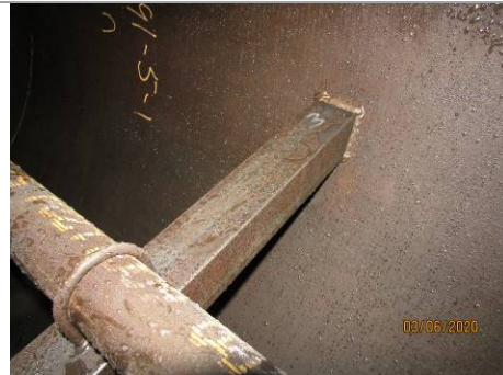
Coil support to shell weld
