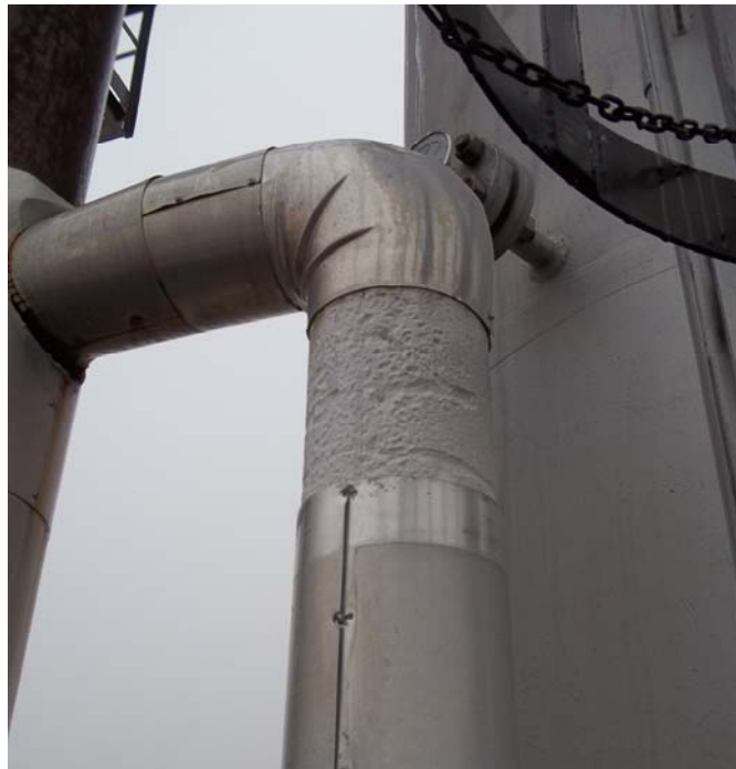
09 exposed insulation
