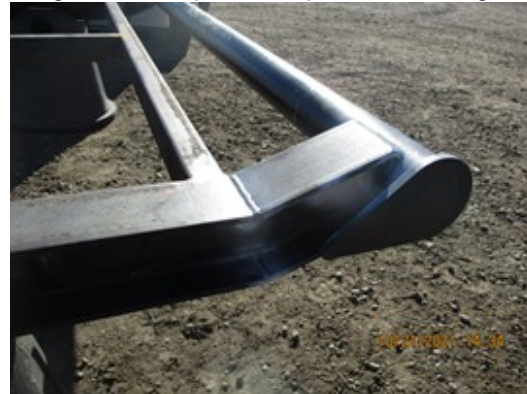
Figure 2: Completed Inspection and Lug Example
