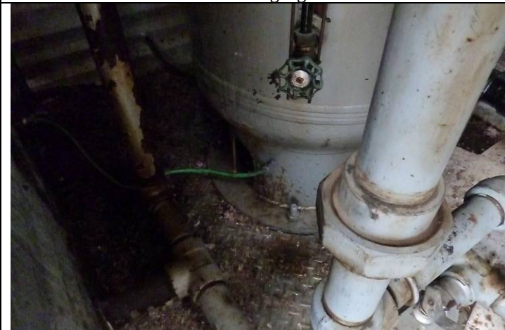
Vessel skirt and ground wire attached
