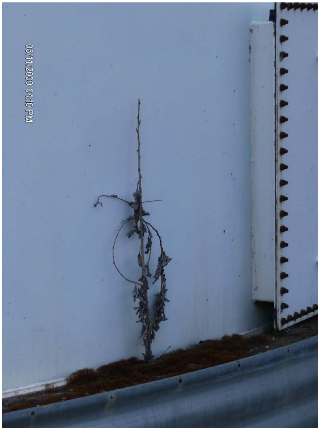
Figure 3_Vegetation Present Around Tank Base_14May09
