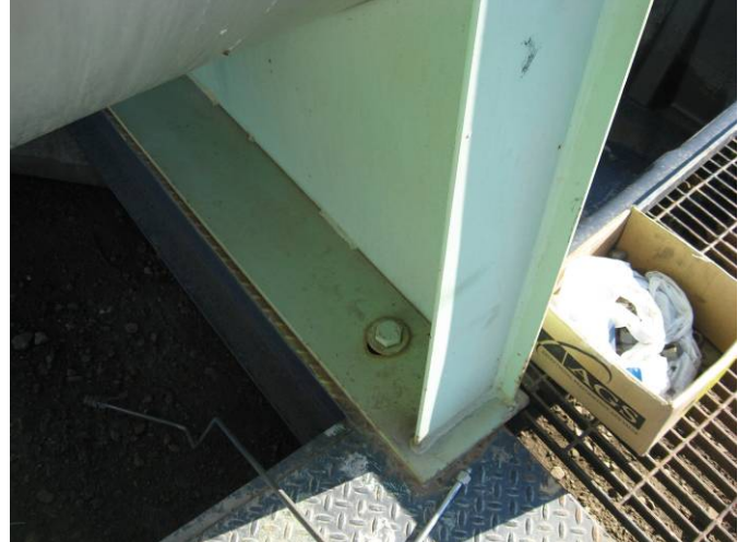
Saddle bolting to skid
