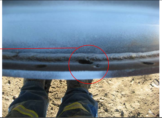
Gouge on inside area of stack attachment flange – to be welded.
