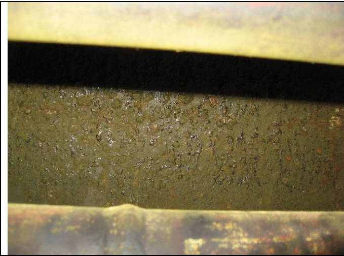
Shell at 12:00 position – light scaling in vapor space – no measureable pitting.
