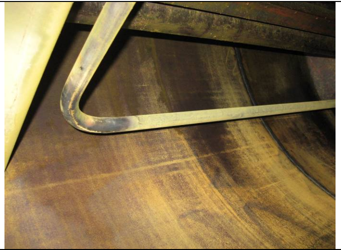
Fuel gas preheat coil
