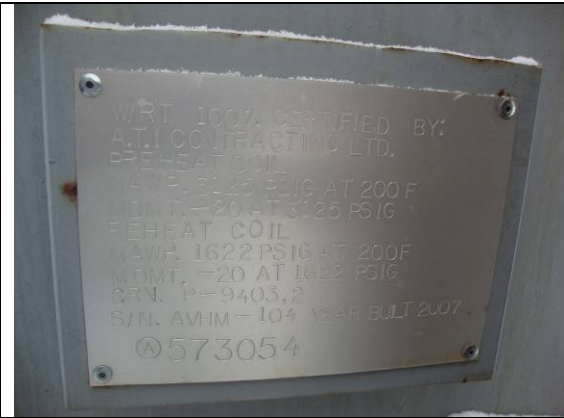
Vessel data plate
