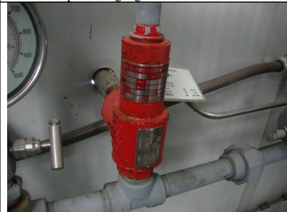
Vessel burner PSV
