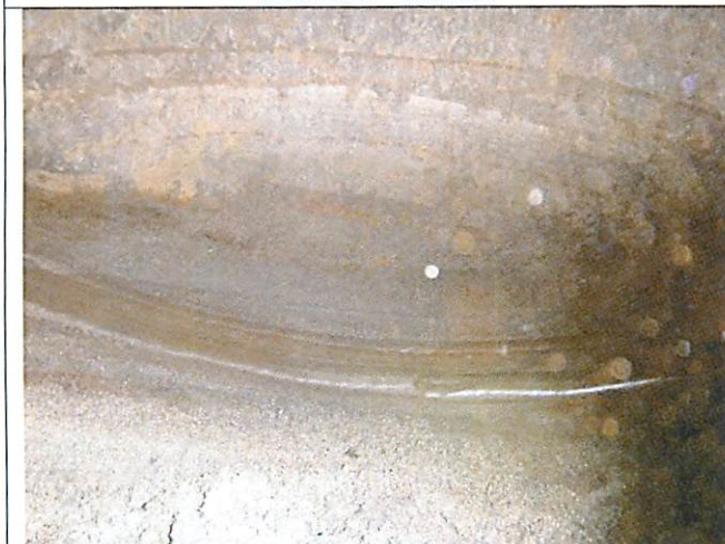
Head to shell weld – no issues
