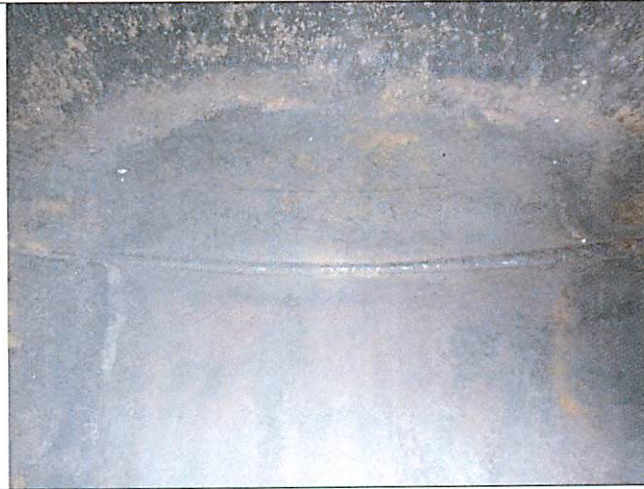
Manway head to shell weld 6:00 position
