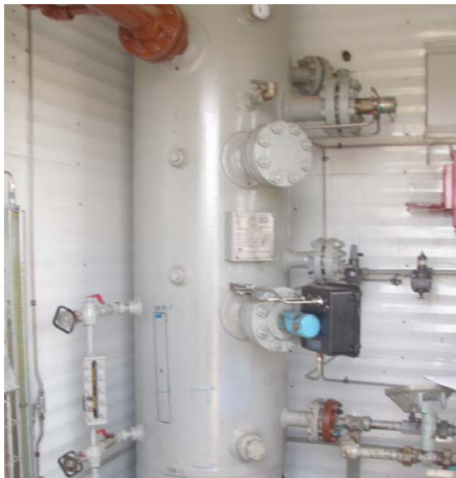
02-A0441749 Overview Inside
