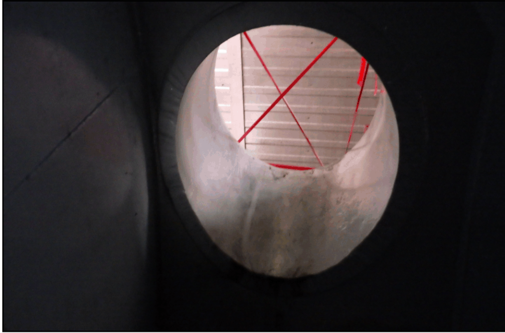
EAST SIDE MANWAY
