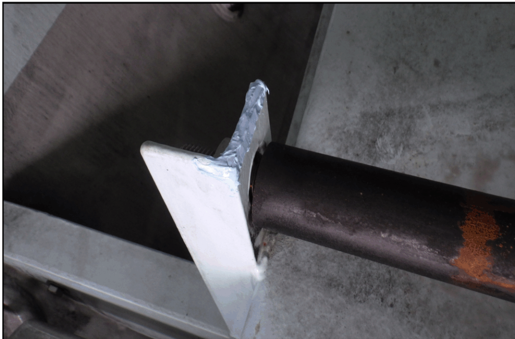
REPAIRED CHIPS ON FIRE TUBE SUPPORTS
