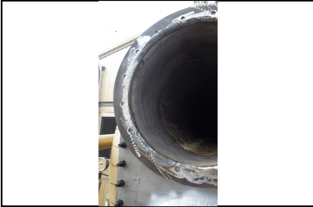
REPAIRED EXHAUST FLANGE
