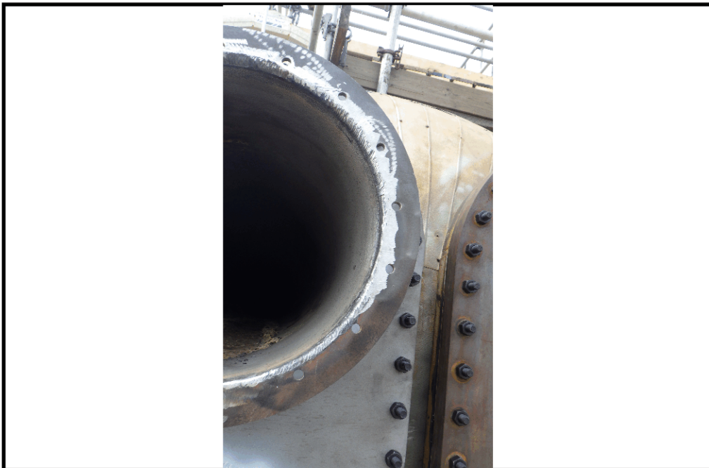
REPAIRED EXHAUST FLANGE
