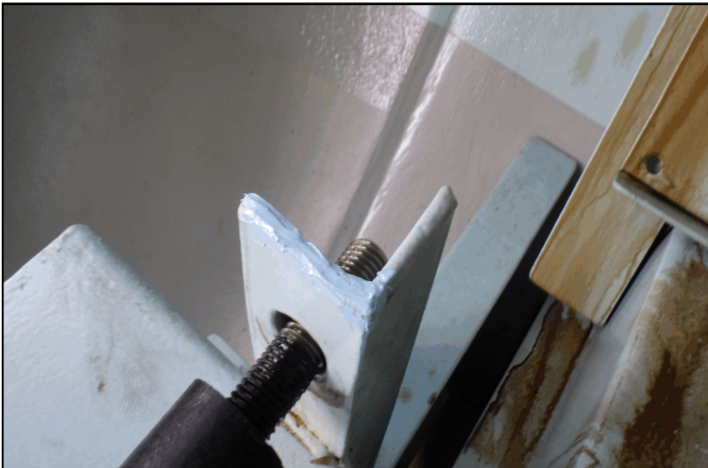
REPAIRED CHIPS ON FIRE TUBE SUPPORTS
