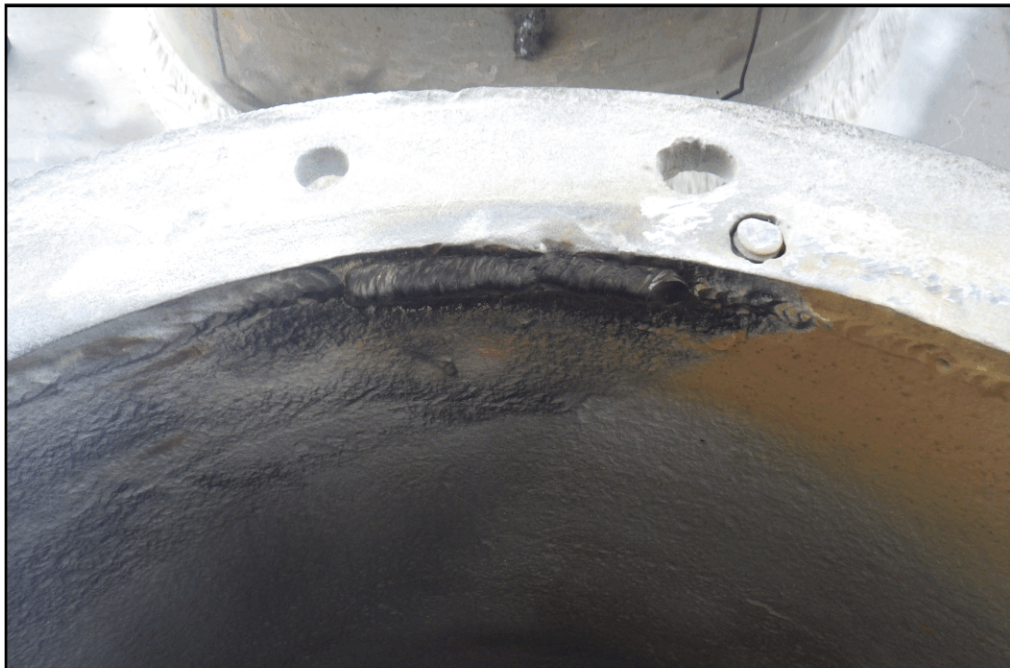
REPAIRED BURNER FLANGE
