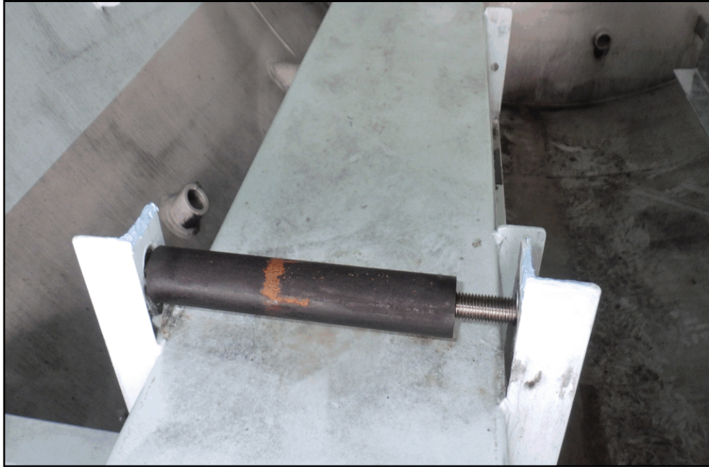
REPAIRED CHIPS ON FIRE TUBE SUPPORTS
