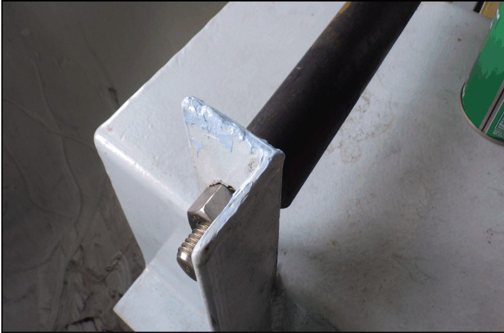
REPAIRED CHIPS ON FIRE TUBE SUPPORTS
