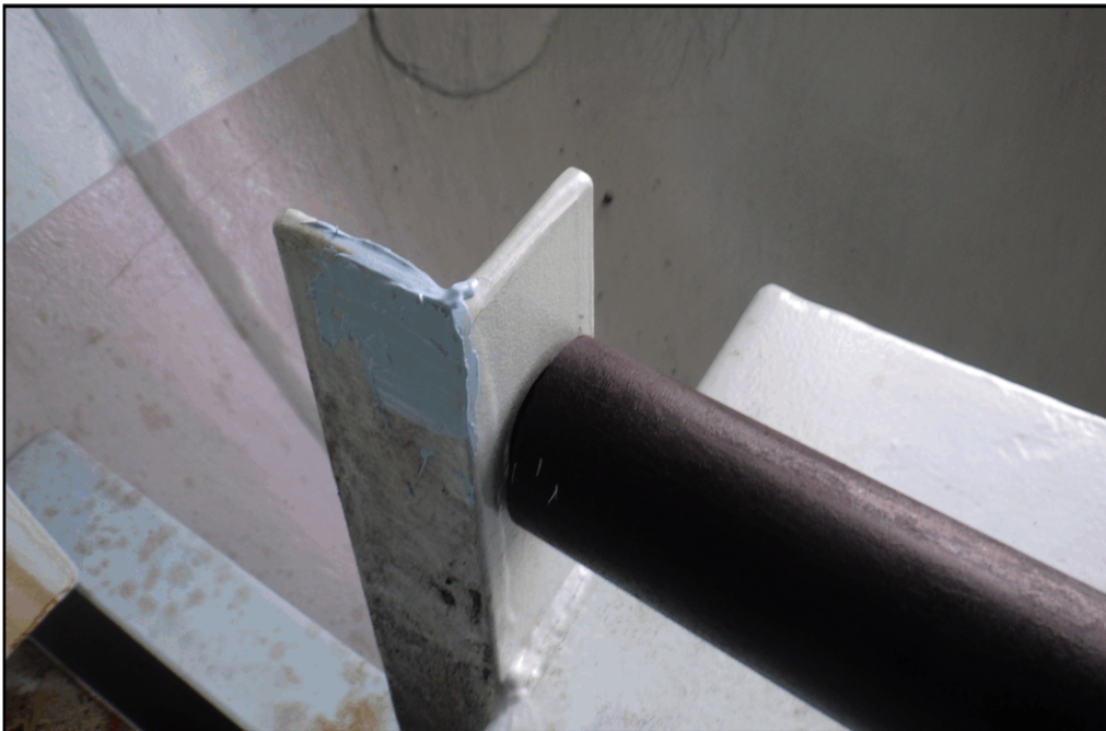
REPAIRED CHIPS ON FIRE TUBE SUPPORTS
