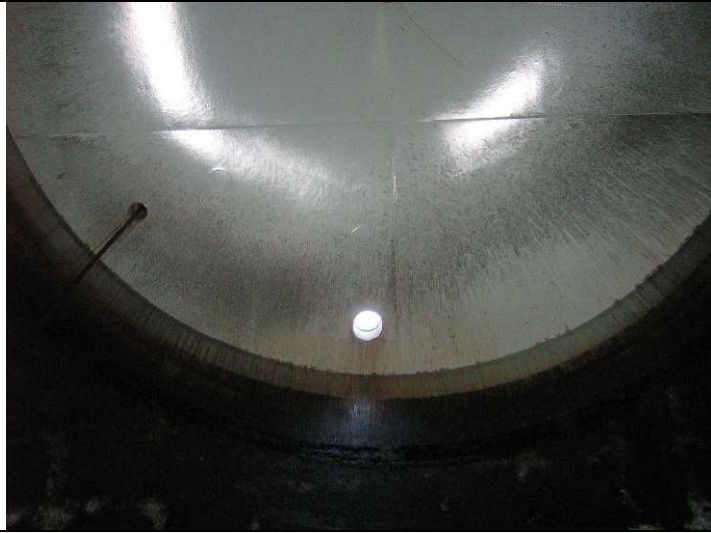
Internal Roof and upper shell
