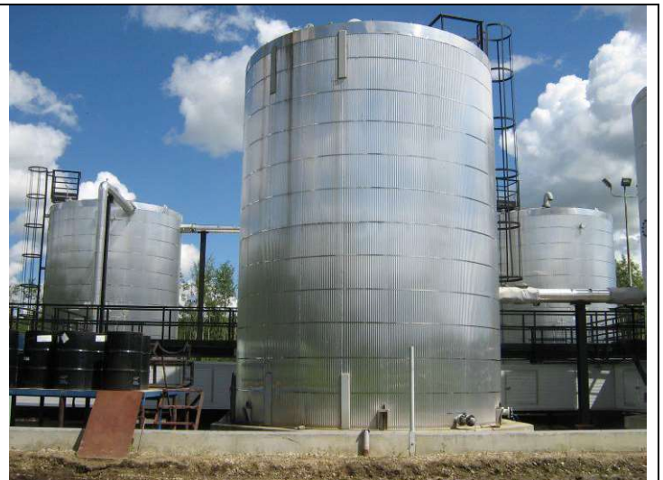
Tank Lot Overview
