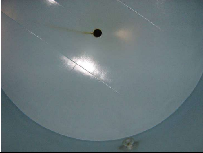
Internal Roof and upper shell
