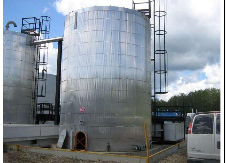
Tank Lot Overview
