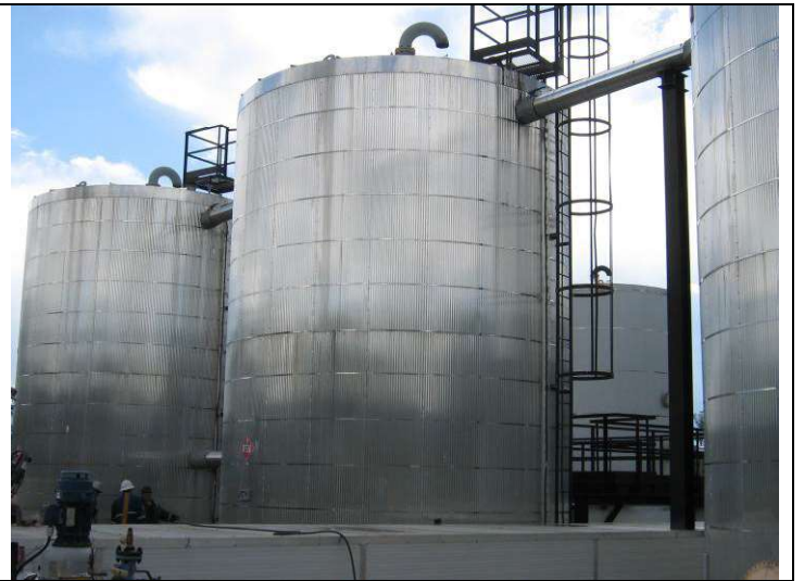
Tank Lot Overview
