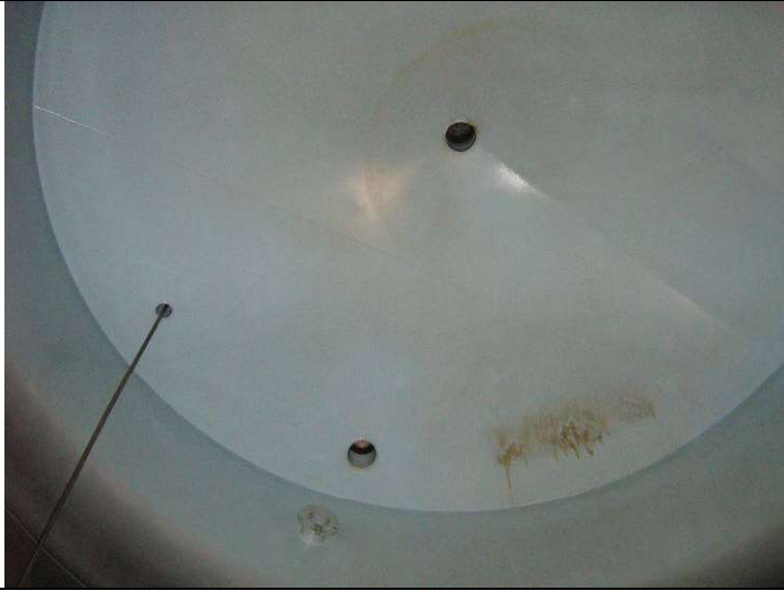
Internal Roof and upper shell
