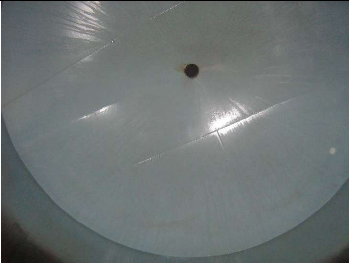
Internal Roof and upper shell
