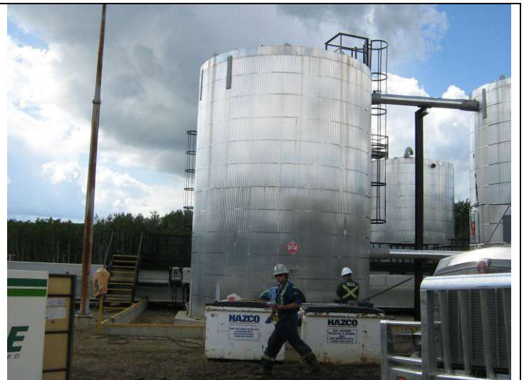
Tank Lot Overview
