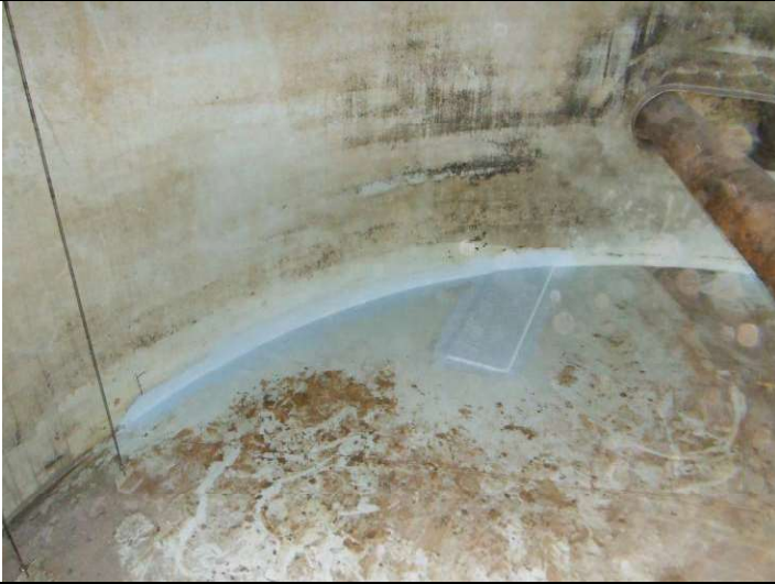
Overview Repair- Bottom patch plate and shell to bottom coating repair.
