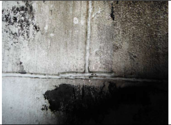
Shell tee weld
