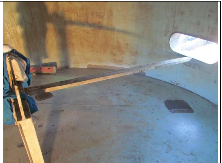
Over view of patched areas – Nov 22.
