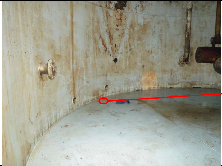
Through hole on bottom
