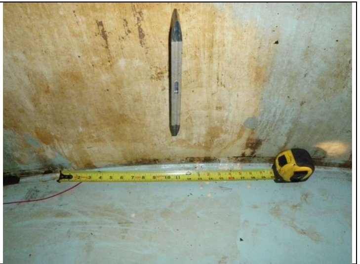
Inward deflection at shell to bottom – 20.0 inches length
