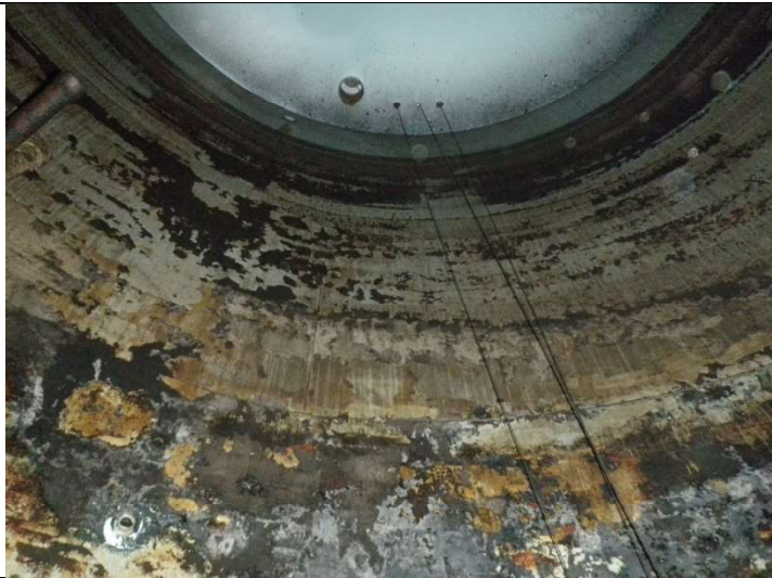
Shell – tightly adhered product scale
