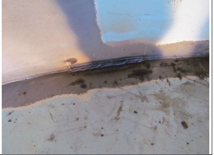
Shell to bottom weld repair.
