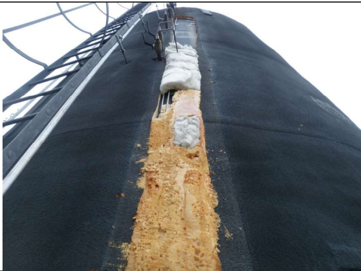
Foam insulation - Open sections
