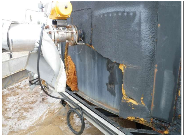
Foam insulation - Open sections
