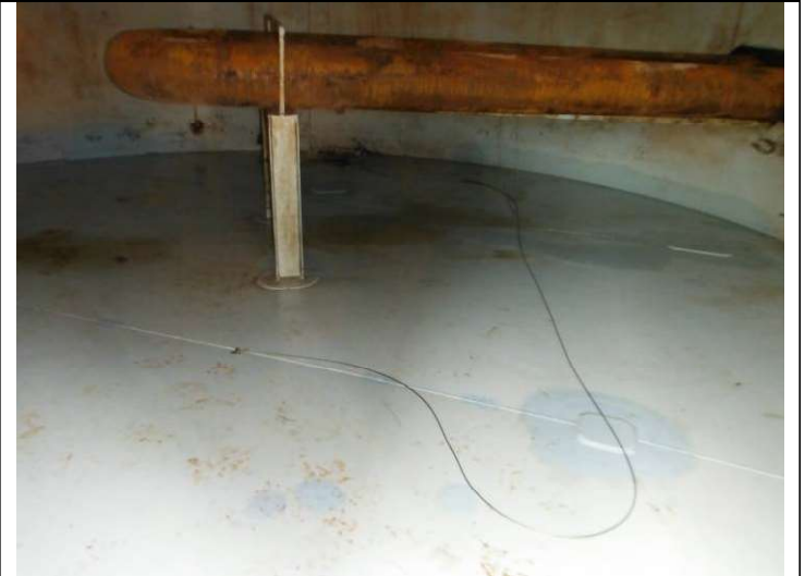
Overview - floor with loose float cable detached.
