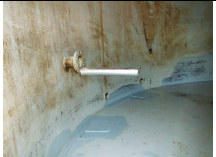
Anode installed
