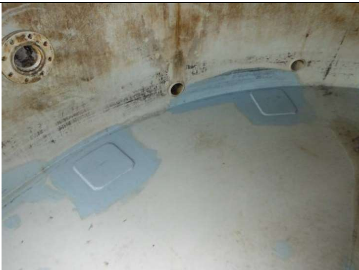
Previously installed patch plates
