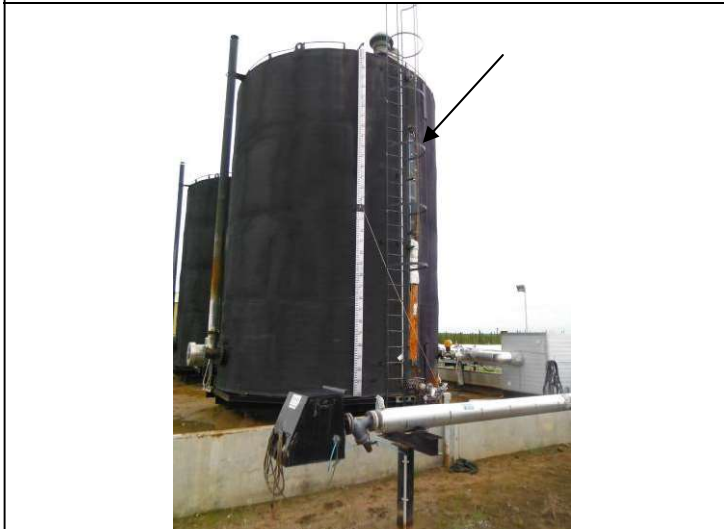
Overview - Tank with large areas of insulation removed
