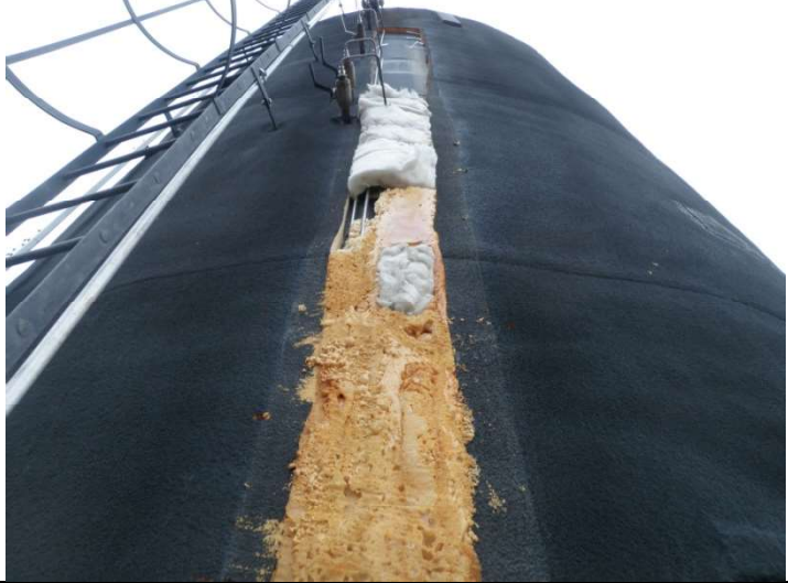
Foam insulation - Open sections
