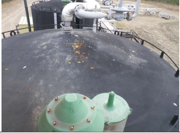
Deck - piping - Vacuum breaker
