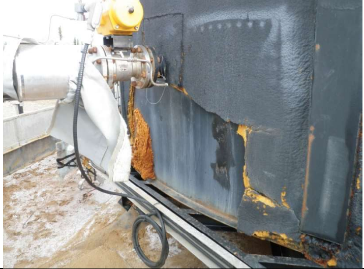
Foam insulation - Open sections
