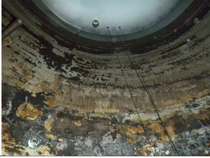
Shell – tightly adhered to product scale
