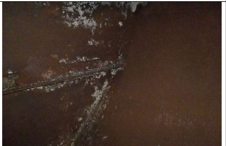
Weir attachment weld
