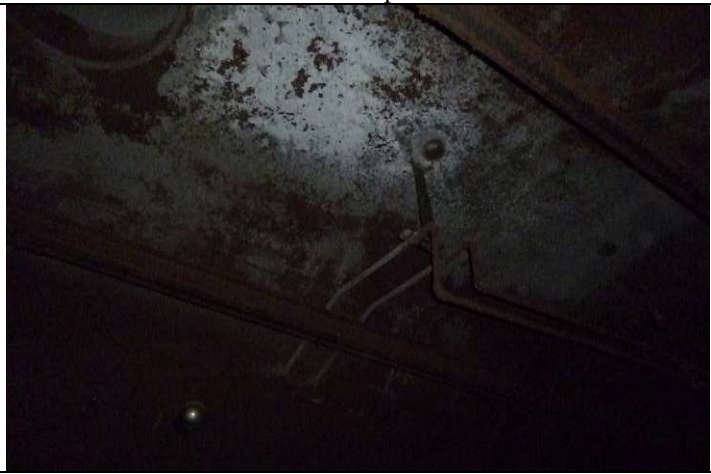
Piping in place
