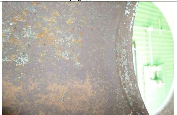
Man way attachment weld
