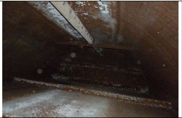
Piping upper shell
