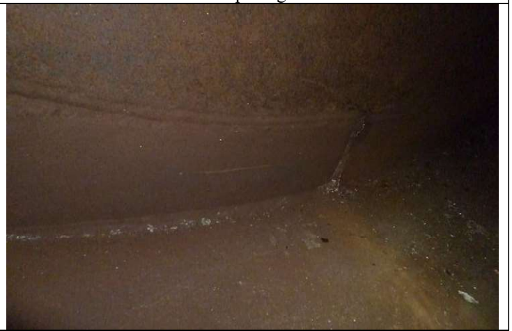
Weir attachment weld
