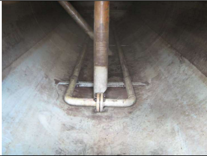
Lower shell overview
