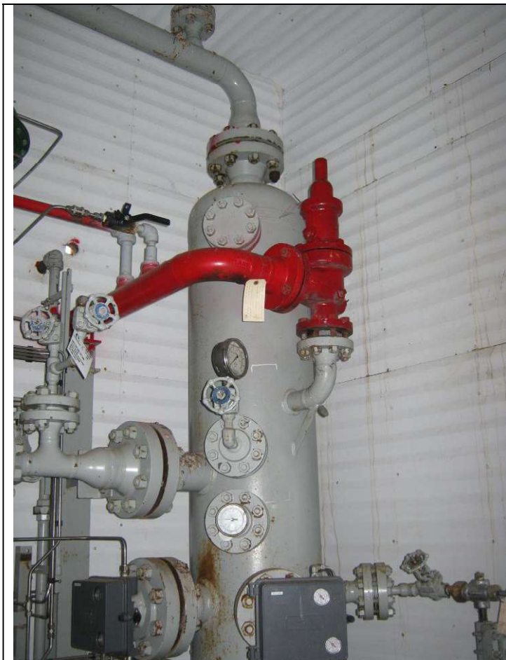
Overview – Vessel upper shell and PSV location
