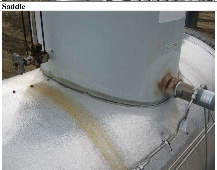
Closure not sealed around expansion tank
