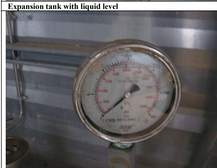
Inlet pressure gauge
