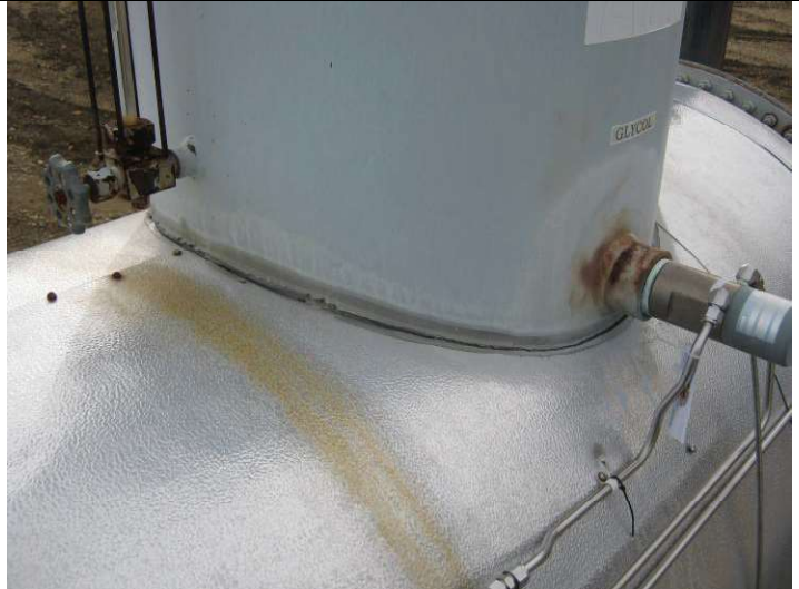
Closure not sealed around expansion tank
