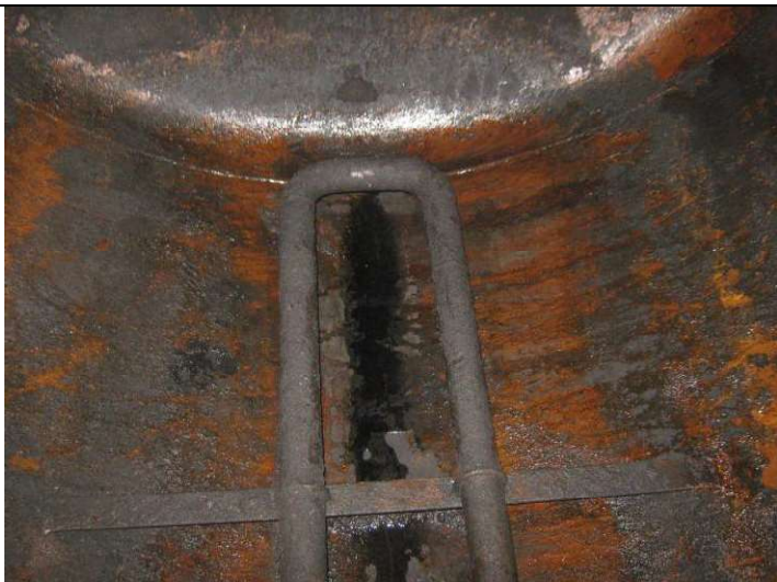
Lower shell and heat medium piping
