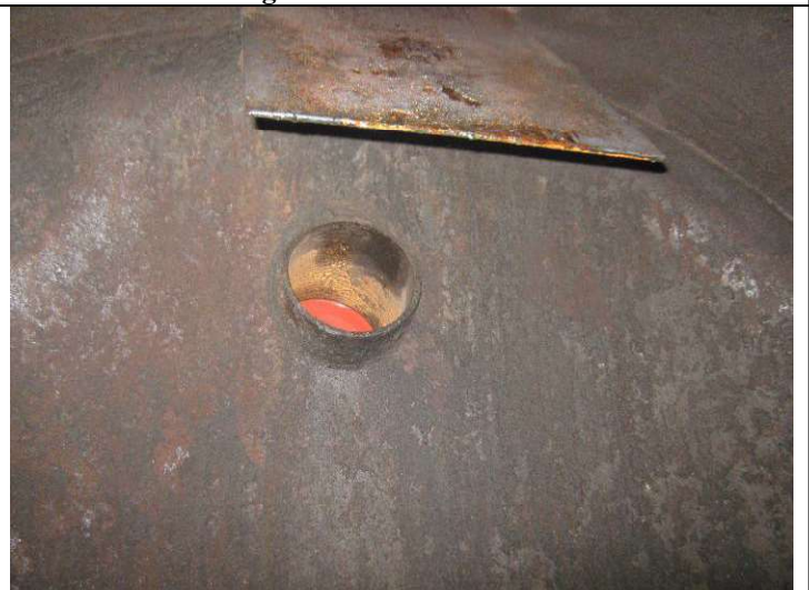
Inlet nozzle and deflector plate
