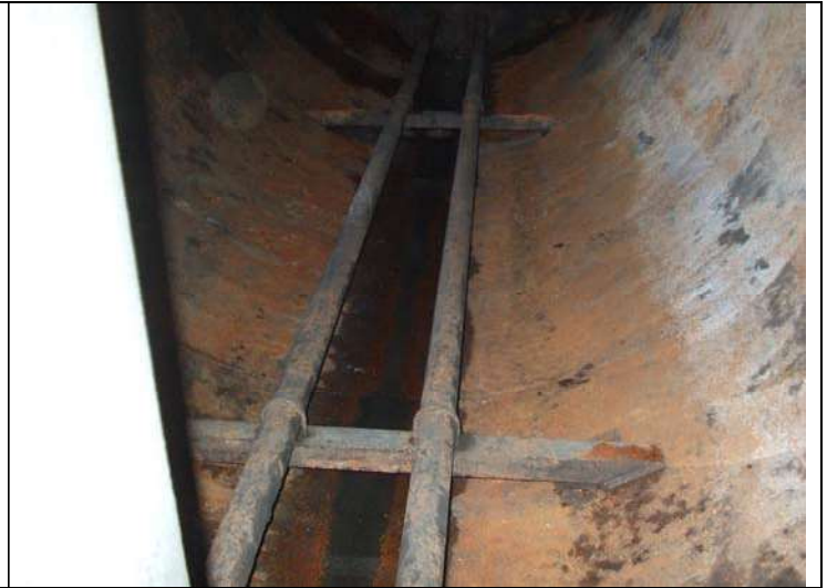
Heater coil overview
