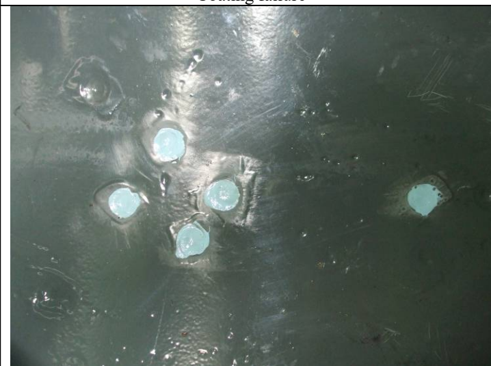
Coating repairs bottom shell / Previous coating repairs
