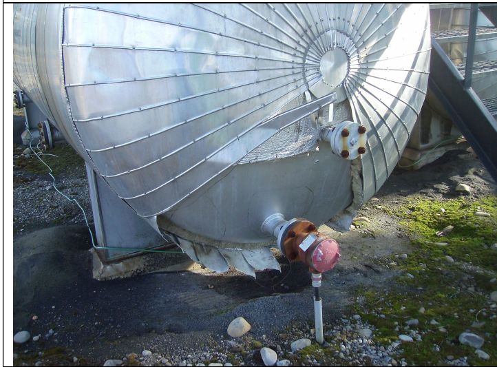
Damaged cladding
