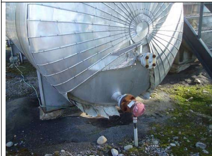
Damaged cladding
