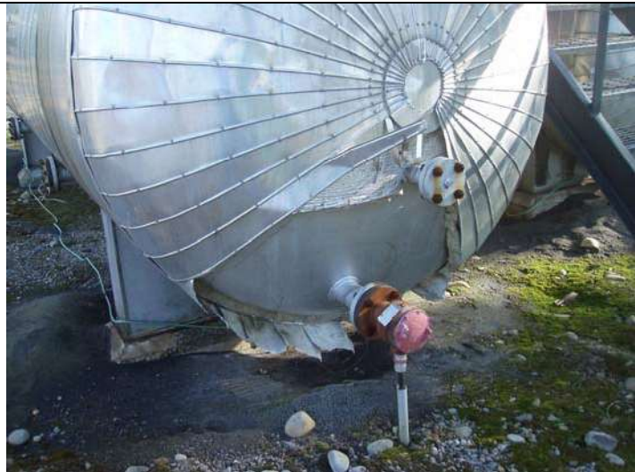
Damaged cladding
