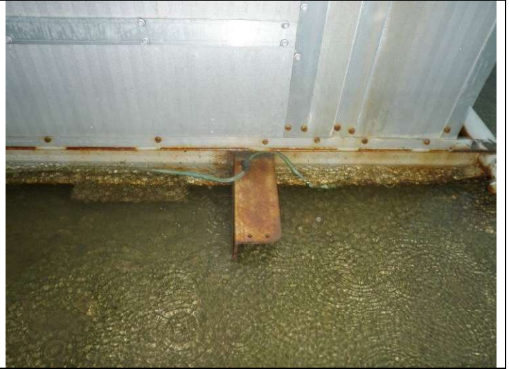
Ground wire attached
