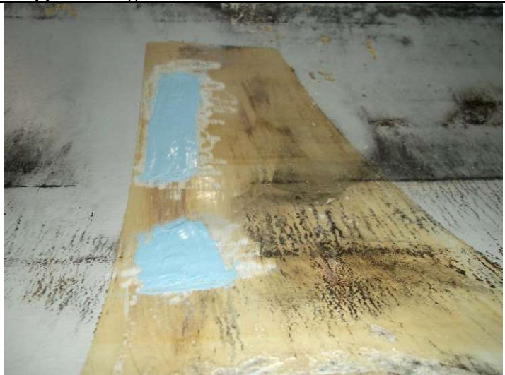
Coating repair at mid shell
