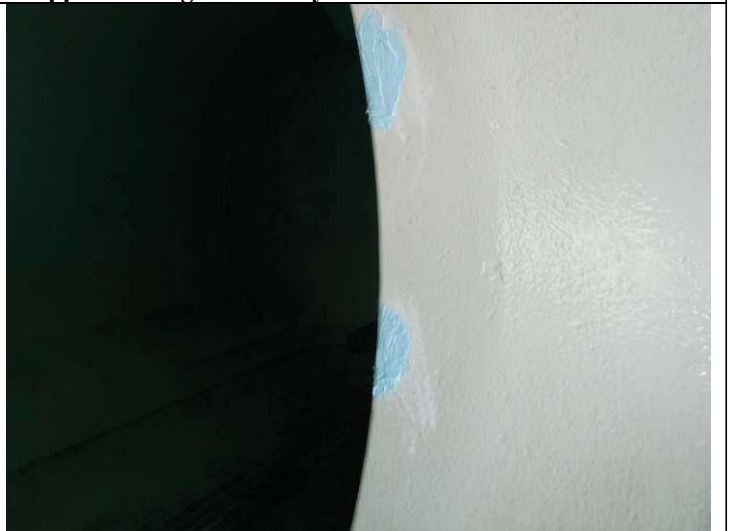
Coating repairs at manway
