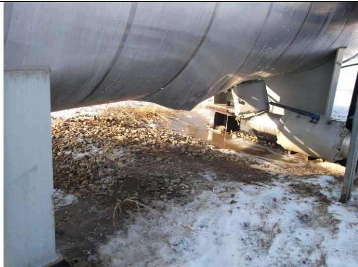
Loose insulation at bottom shell
