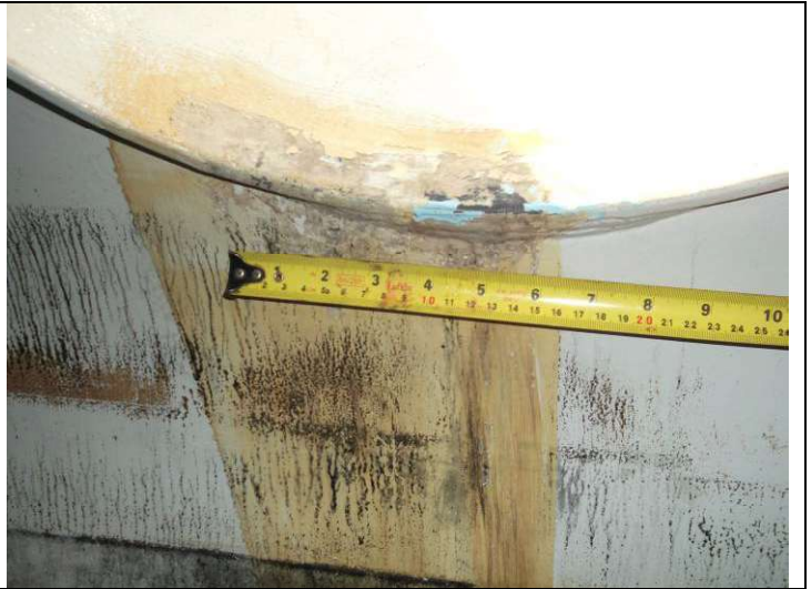
Previous coating repair – no exposed metal
