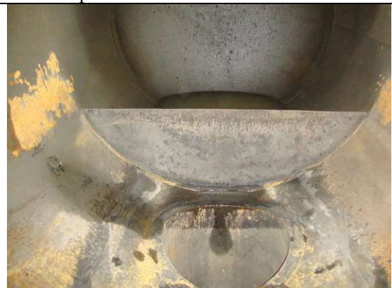
Overview of north head, weir and boot
