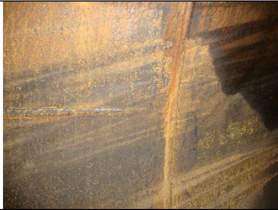
Shell tee weld
