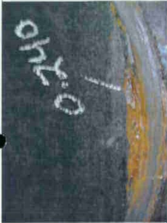
Corrosion at manway cover
