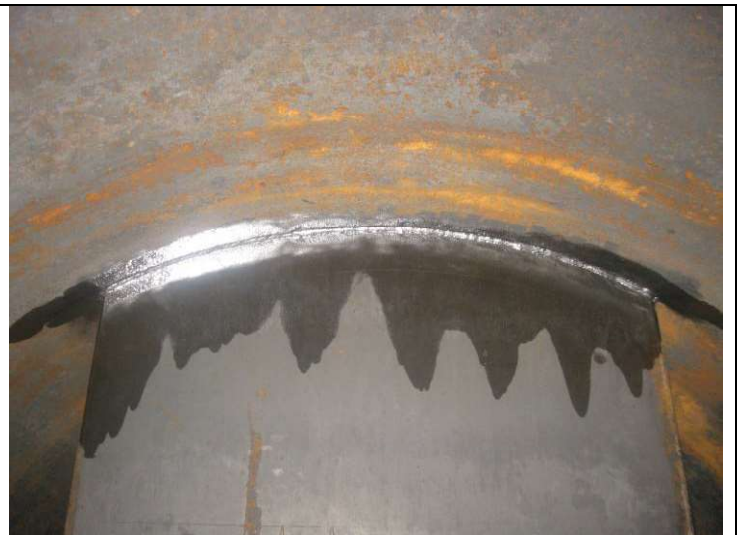
Demister pad weld to shell
