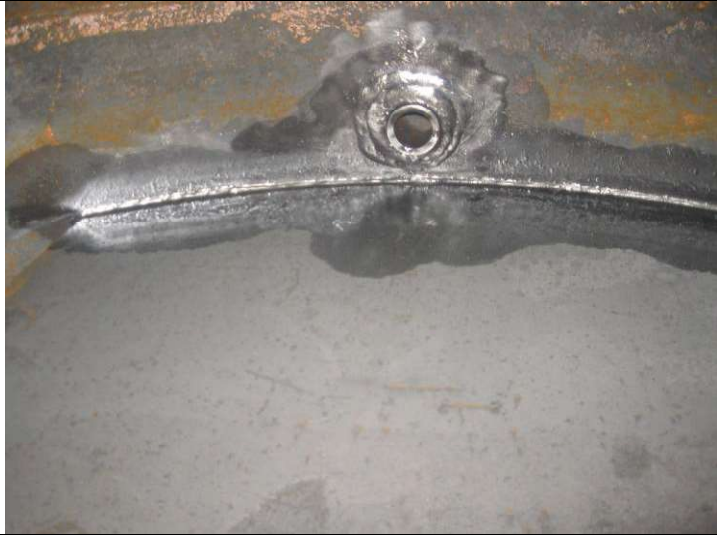
Nozzle by Demister pad support weld to Shell
