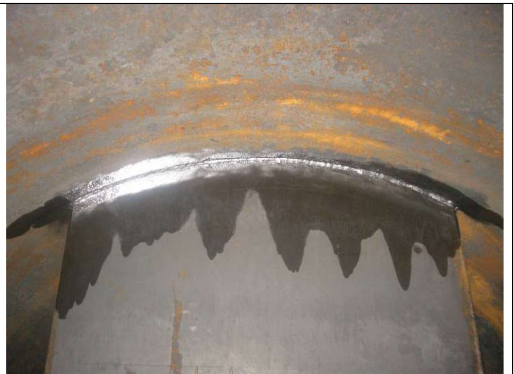
Demister pad weld to shell
