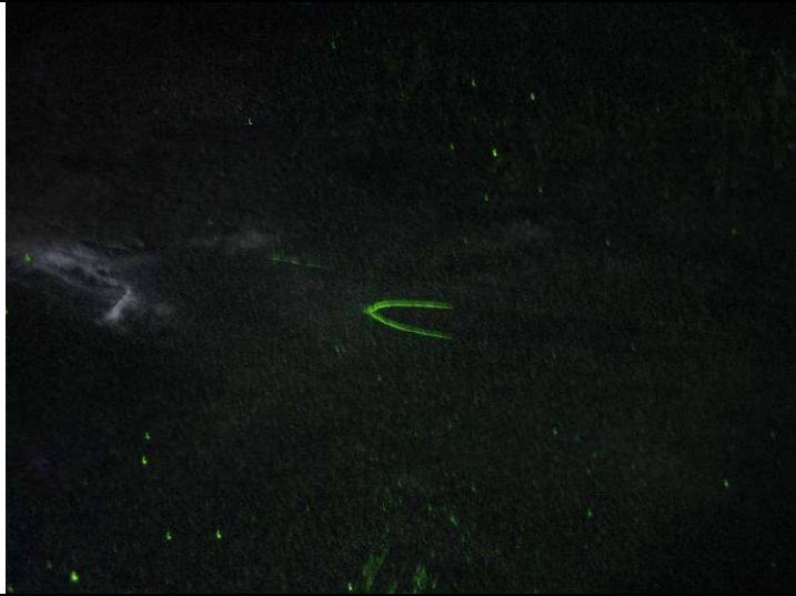
View of crack above tee intersection
