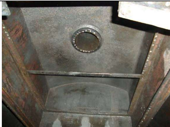
Demister pad support frame and top shell
