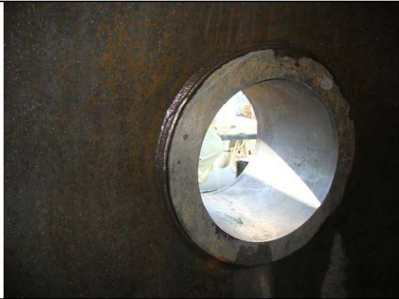
Man way attachment weld to vessel
