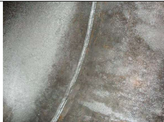
Head to shell weld
