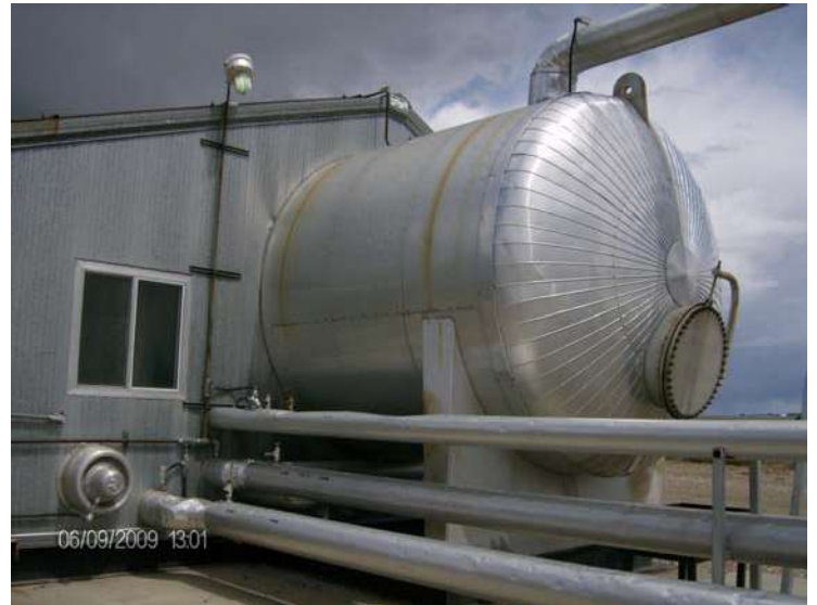
Grand Forks-FWKO Outside Bldg.
