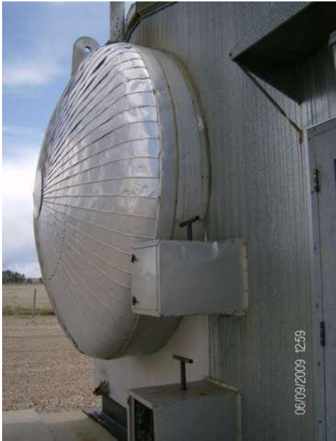
Grand Forks-FWKO Outside Bldg.
