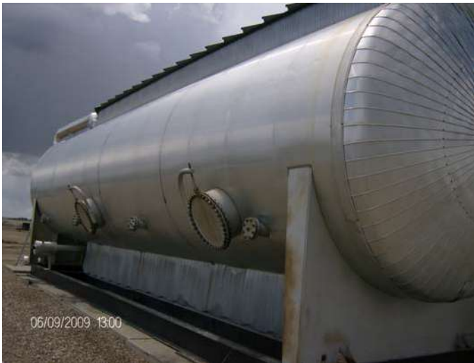
Grand Forks-FWKO Outside Bldg.
