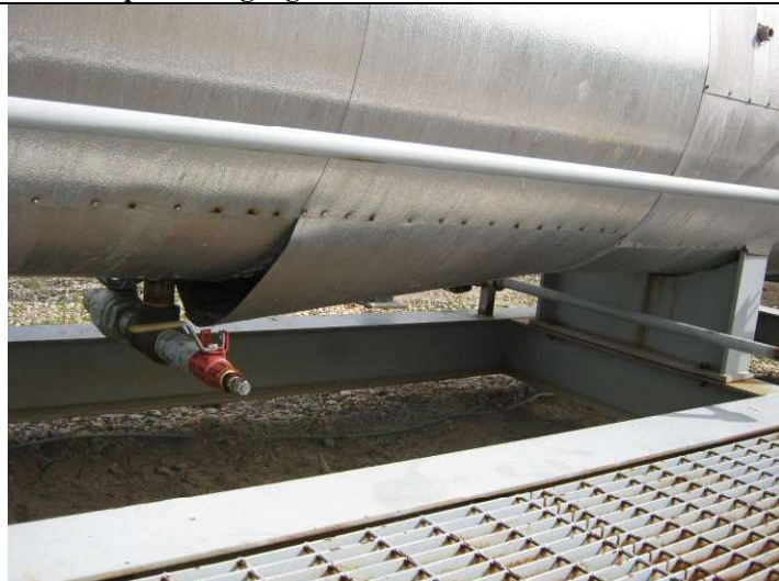
Bottom shell - Loose cladding and wet insulation
