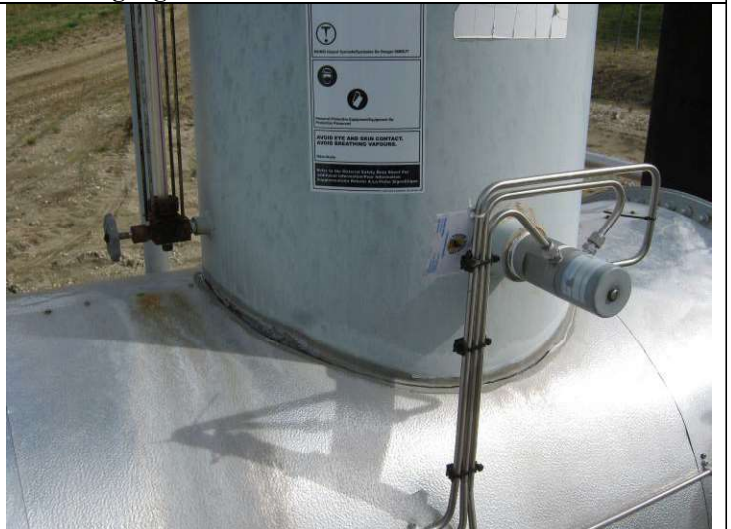
Closure not sealed around expansion tank
