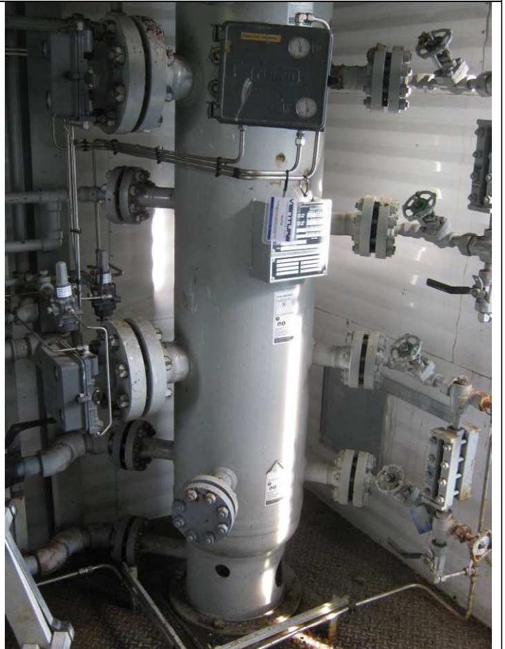
Overview – Vessel lower shell
