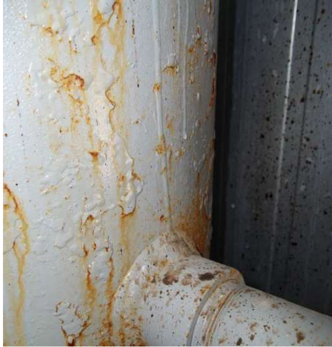
05 paint deterioration
