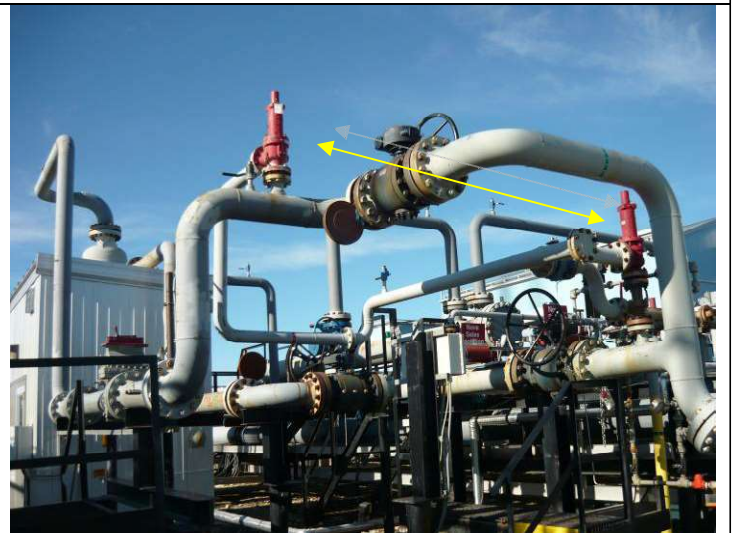
Two PSV's on the same sales line (left=1 right =2) second PSV was recorded on excel list.
