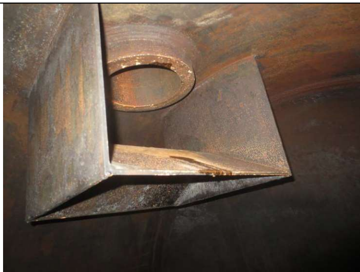
Inlet deflector is in good condition.
