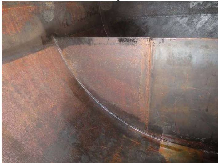
Weir is in good condition.
