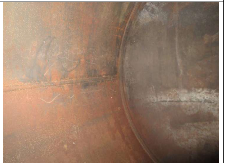
Shell is in good condition with no corrosion or pitting.
