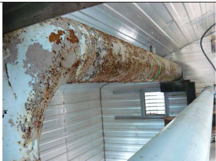
Outlet Piping (Paint)
