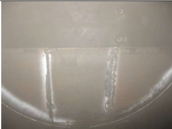
Weir Plate to Shell
