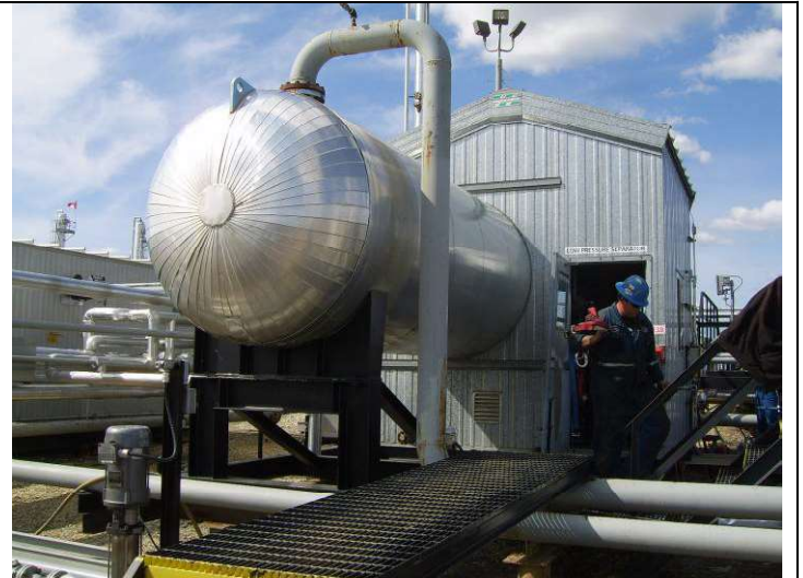
Vessel Overview Outside Building
