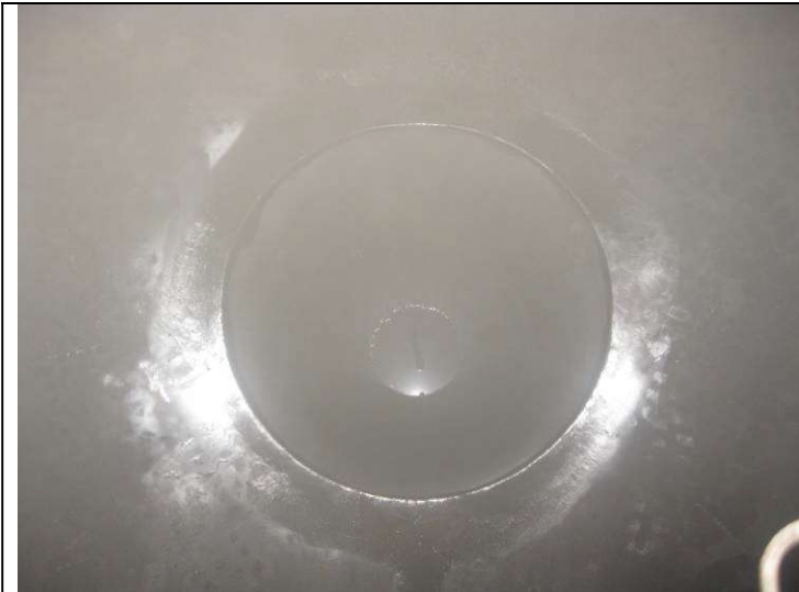
Bottom Boot to shell weld
