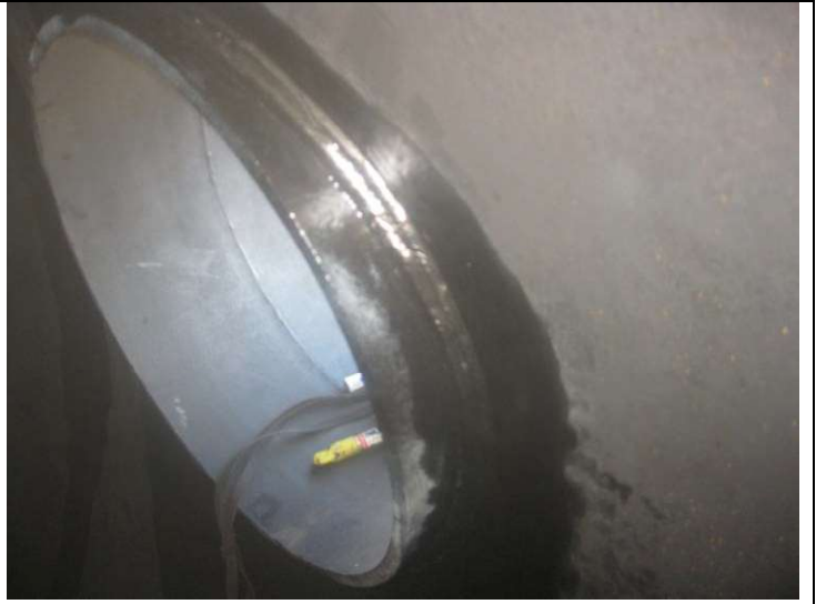
Manway weld to shell
