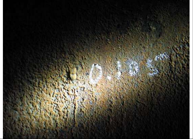
Pitting at bottom of shell.
