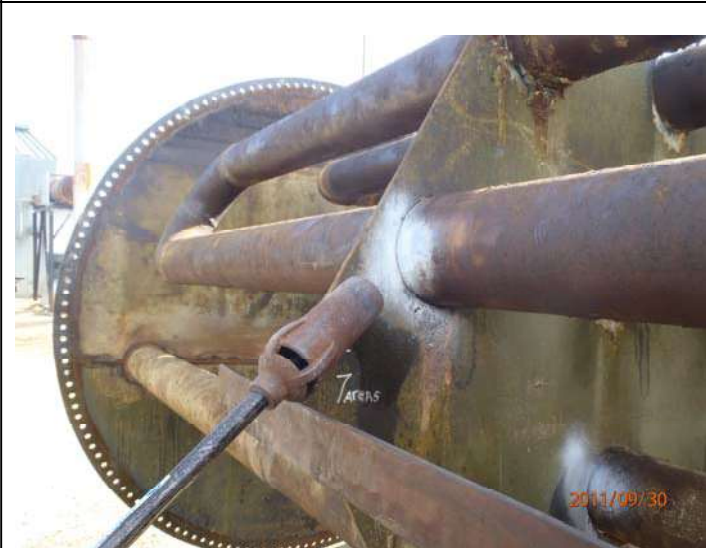
Preheat and MPI on locations before welding
