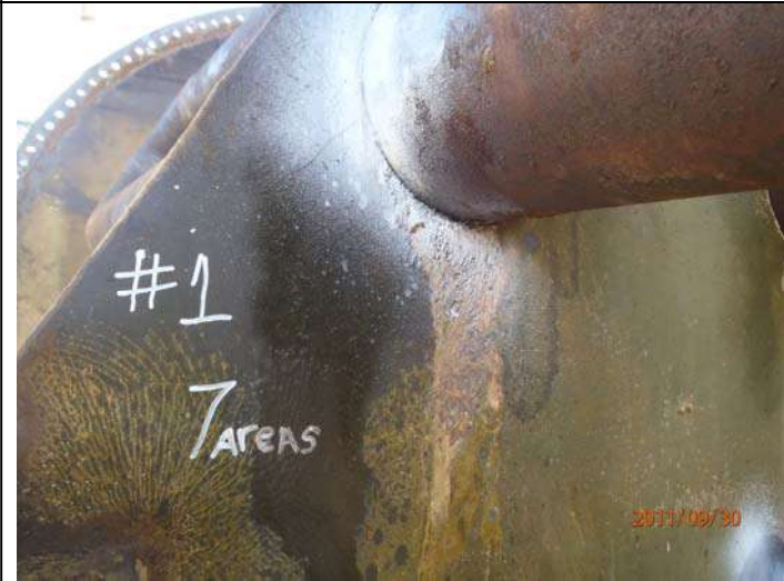
7 Tack Weld Locations on each Divider
